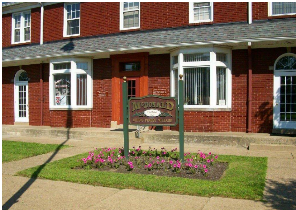
Village of McDonald Administration Building
