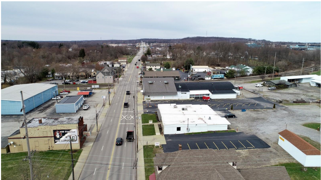
Hubbard Aerial View
