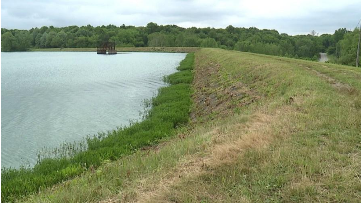
Upper Girard Lake Dam – online photograph
