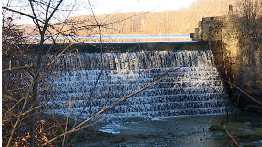
File photo of Coalburg Lake Dam
