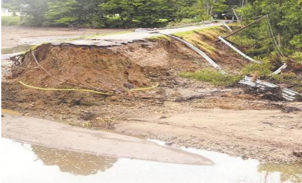
Photo from Star Beacon, taken by Warren Dillaway regarding Kinsman Dam Incident where road and bridge washed out after heavy rain.
