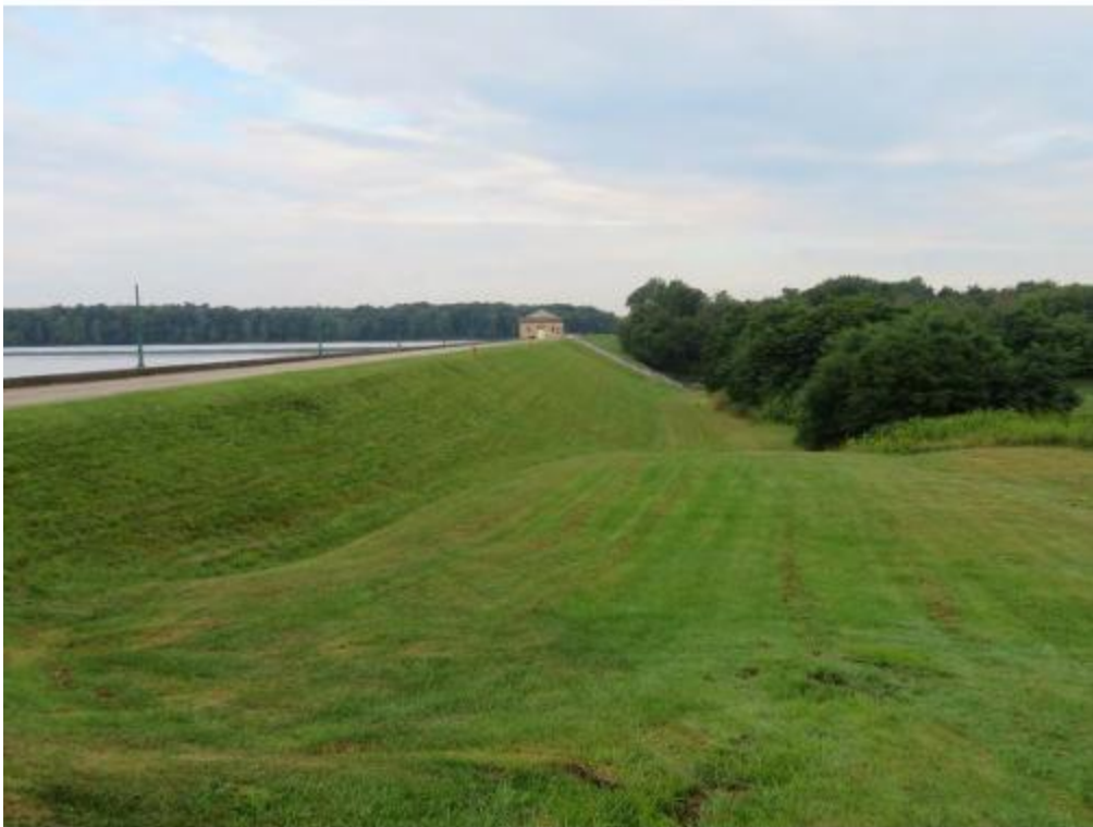
Figure 7. TRU-02944-23: Embankment, looking west. Photos taken from FEMA Rehabilitation Plan
