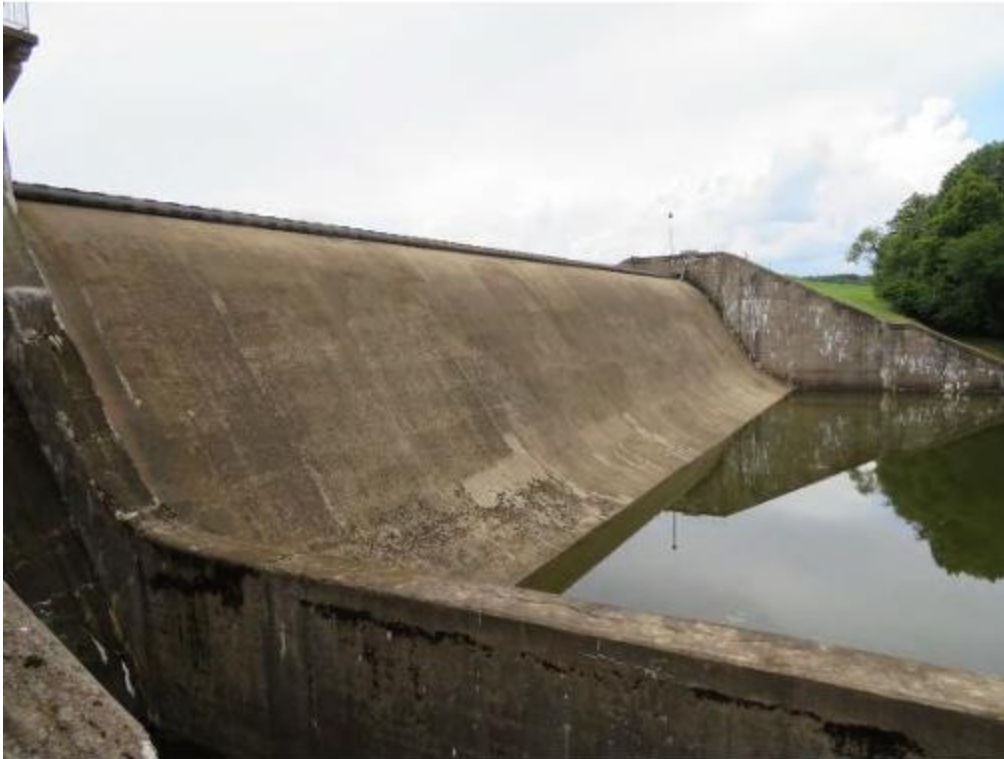
Figure 6. TRU-02944-23: Mineral Ridge Dam, looking southwest.
